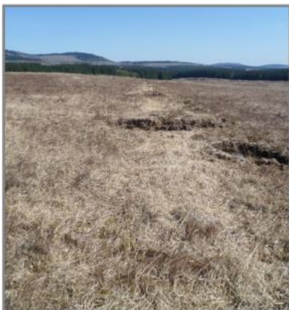
Figure 2 Hill drain blocked with peat dams at Cairnsmore of Fleet
